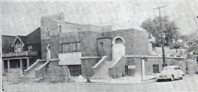
FIRST UNIT OPENED DECEMBER 1946
